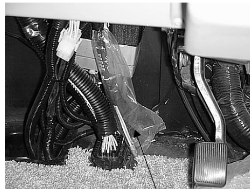
CB Wires (in plastic sheath)
