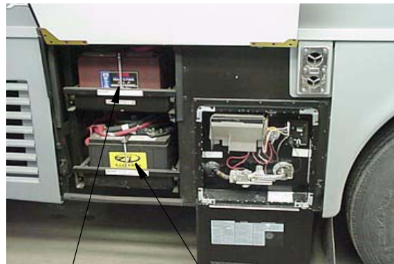
House Batteries Chassis Batteries
