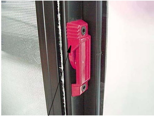
Pull latch outward to slide window open
