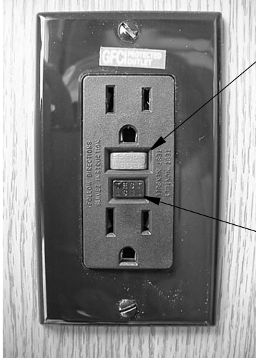
GFCI Outlet (Ground Fault Protector)
