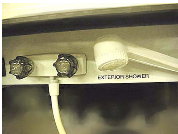
Exterior Shower/Wash Station (Typical)
