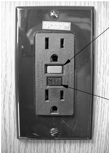
GFCI Outlet (Ground Fault Protector)
