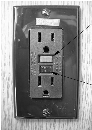
GFCI Outlet (Ground Fault Protector)
