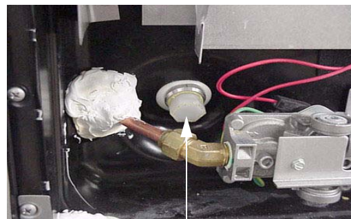
Water Heater Drain Plug (Remove with socket)
