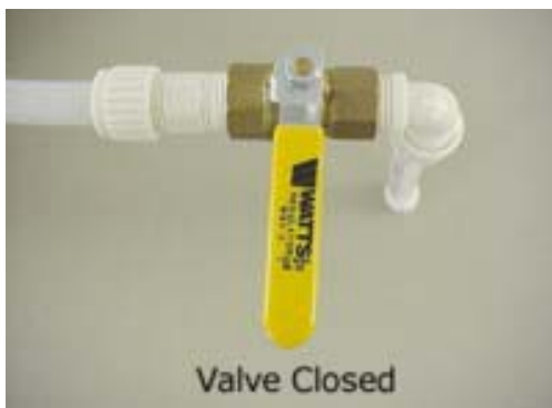
Water Tank Drain Valve (Located in first passenger side compartment) -Typical View
