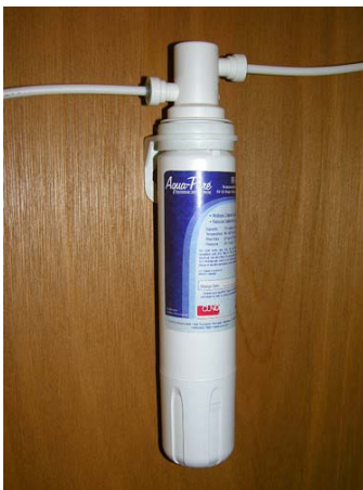
Water Filter Assembly (Located below Galley Sink)
