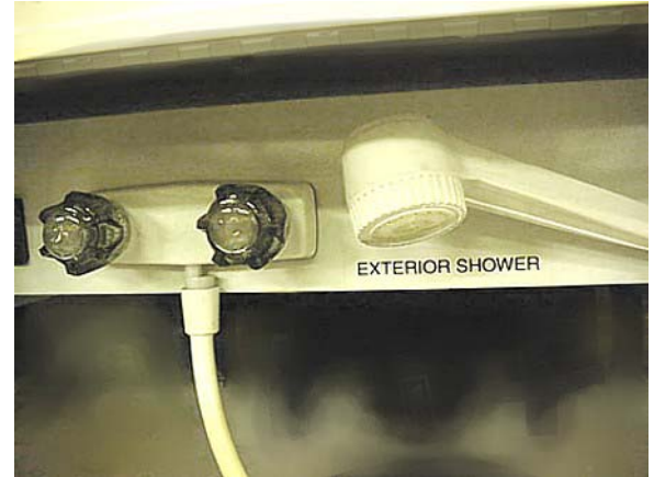
Exterior Shower/Wash Station -Typical View
