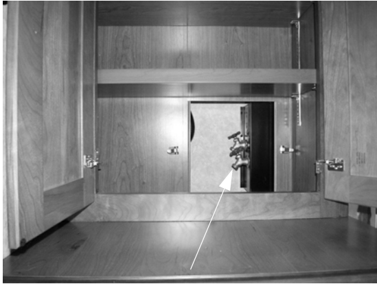
Water Supply Faucets -Typical Installation
