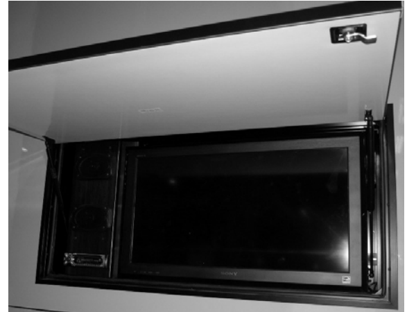
Exterior Entertainment Center -Typical View
