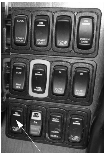
Chassis Battery Disconnect Switch (Located near entrance door) -Typical View
