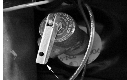
Pressure-Temperature Relief Valve
