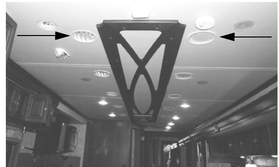
Supply/Return Air Vents (Located throughout the ceiling of the coach) * View looking to rear of coach
