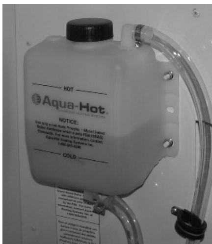
Expansion Fill Tank
