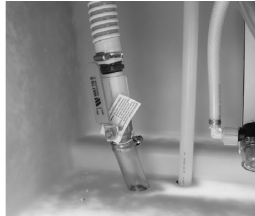
Water Tank Drain Valve -Typical installation shown
