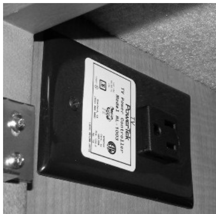
Front TV Ignition Switch Interlock -Typical View
