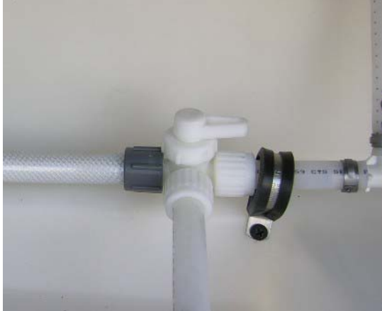
Waterline Drain Valve -Typical installation shown
