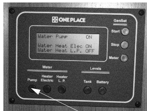
Water Pump Switch
