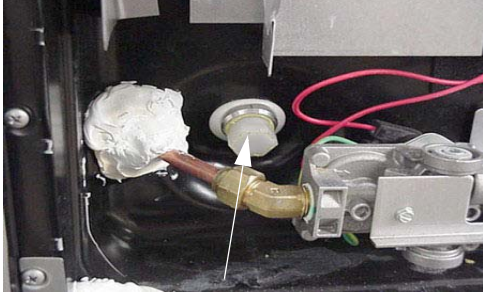
Water Heater Drain Plug (Remove with socket)
