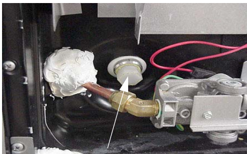
Water Heater Drain Plug (Remove with socket)
