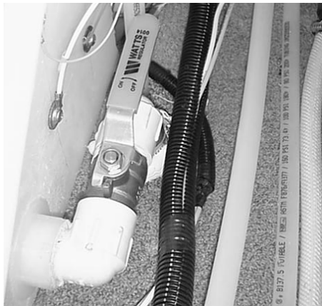
Water Tank Drain Valve -Typical installation shown
