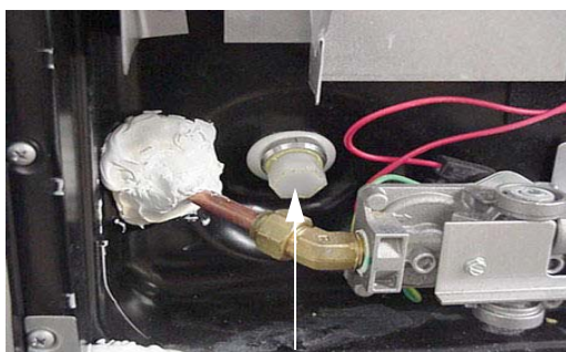
Water Heater Drain Plug (Remove with socket)
