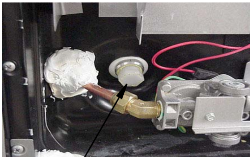
Water Heater Drain Plug (Remove with socket)
