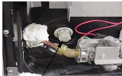
Water Heater Drain Plug (Remove with socket)
