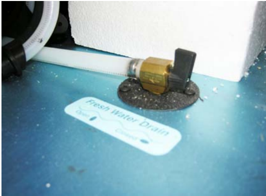
Water Tank Drain Valve -Typical Installation
