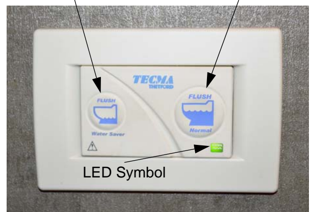
Wall Switch/Controller (Located on wall near toilet)
