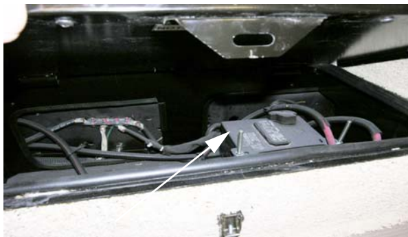
Chassis Battery (located beneath entrance step) -Models 38Q and 37F
