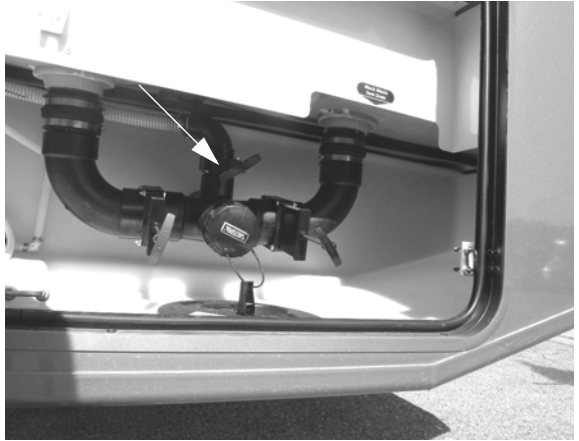
Black Waste Tank Drain Valve #2 (Front) (Located in water service center) -Typical View
