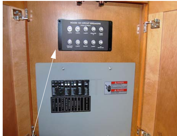
House 12-Volt Circuit Breakers (Models 35B and 35F) -Typical View
