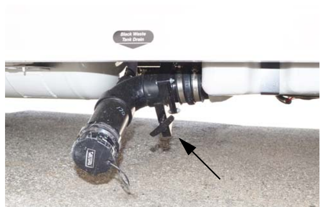
Black Waste Tank Drain Valve (Located beneath coach on mid-driver side) -Typical View
