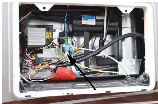
Ice Maker Water Supply Connection -Typical View
