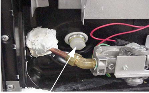
Water Heater Drain Plug (Remove with socket)
