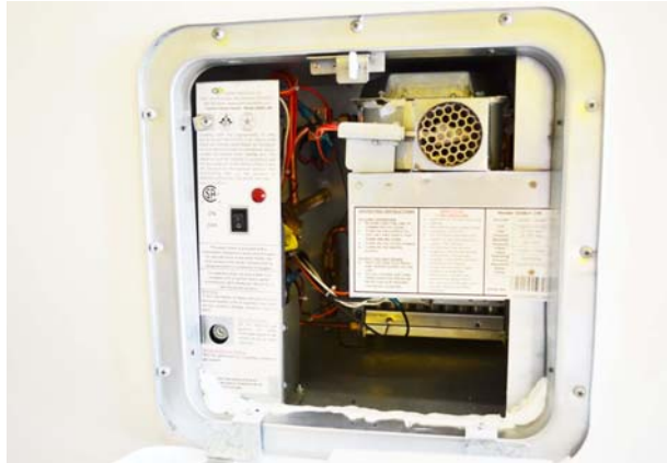
Water Heater Exterior Service Access -Typical View
