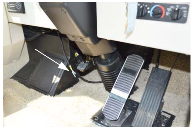
CB Power Wires -Typical View
