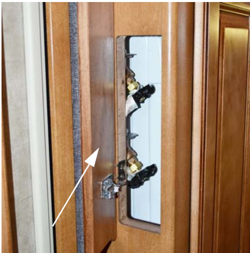
Water Supply Faucets (Located behind access door rear of the washer/dryer cabinet.) * Model 33C shown
