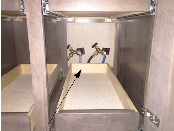
Water Supply Faucets (Located inside pantry cabinet above washer/ dryer, remove panel to access) *Model 36Z shown
