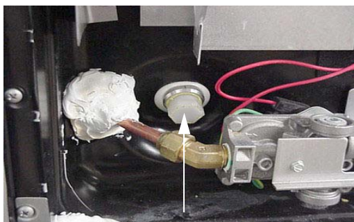
Water Heater Drain Plug (Remove with socket)
