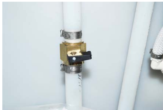
Water Tank Drain Valve -Typical installation shown
