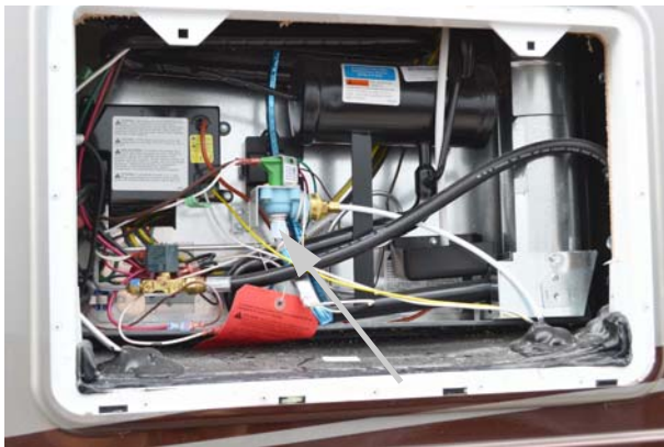
Ice Maker Water Supply Connection -Typical View
