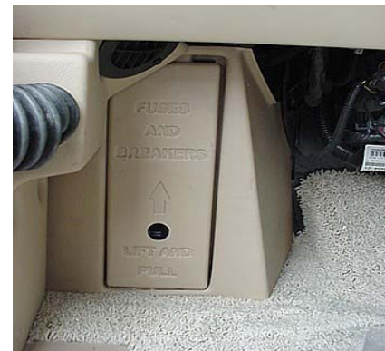
Automotive 12-Volt Circuit Breakers and Fuses (Located beneath left end of dash) -Typical View
