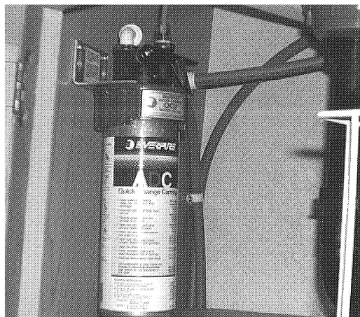
Water Filter Assembly - Below Galley Sink
