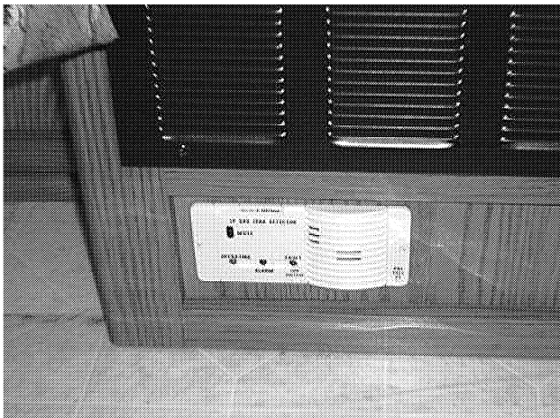
LP Gas Leak Detector
