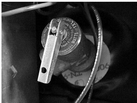
Lift straight out to open P-T valve
