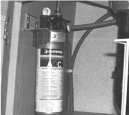
Water Filter Assembly - Below Galley Sink
