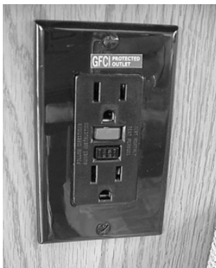
GFCI Outlet (Ground Fault Protector)
