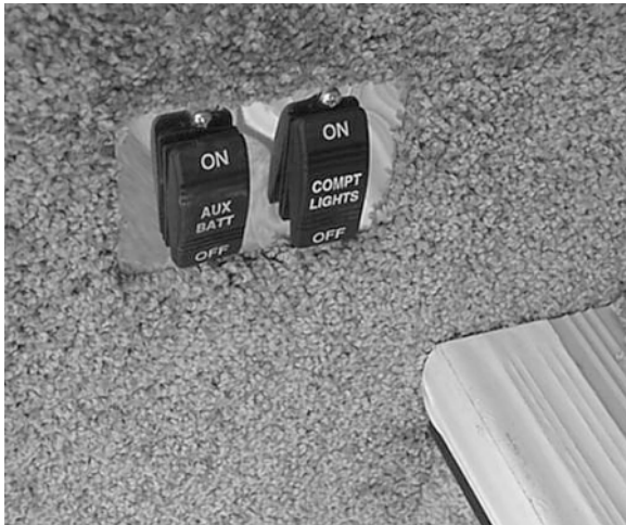
Aux. Batt. Switch (Near entrance door)
