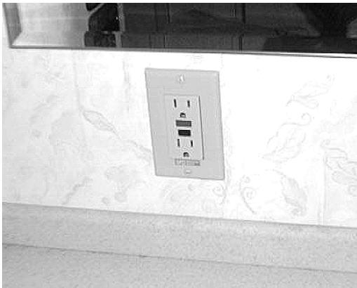
Ground Fault Circuit Interrupter (GFCI)
