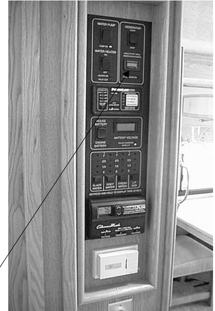
Generator Switch and Hourmeter
