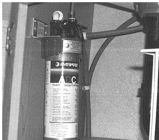
Water Filter Assembly - Below Galley Sink
