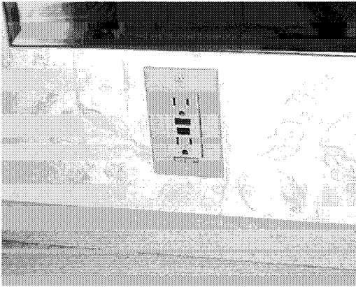
Ground Fault Circuit Interrupter (GFCI)
