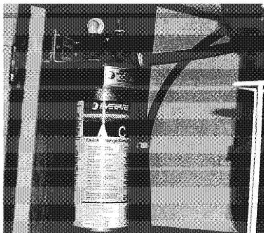
Water Filter Assembly - Below Galley Sink
