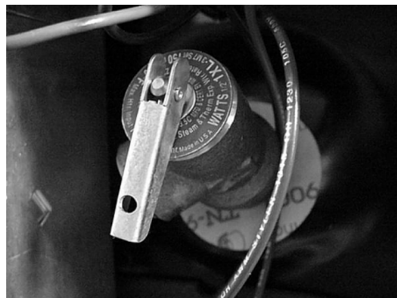
Lift straight out to open P-T valve
