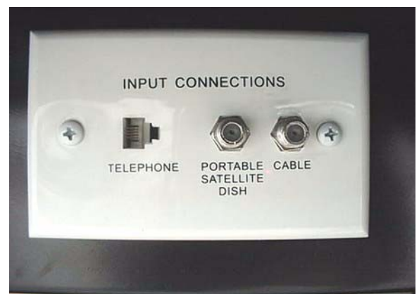
Exterior Connection for Satellite Dishes and Cable TV (In Water Center or Shoreline Compartment)
