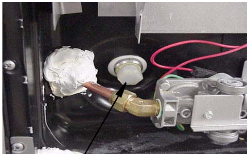
Water Heater Drain Plug (Remove with socket)
