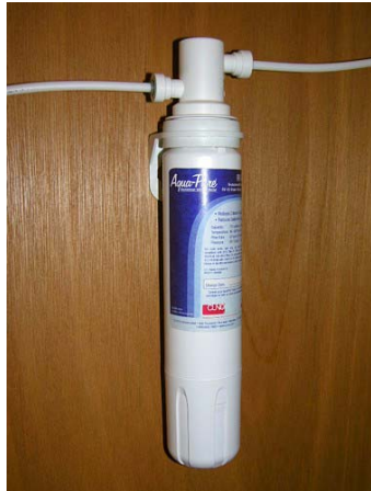
Water Filter Assembly below Galley Sink (Located below galley sink) * Typical View - your coach may vary
