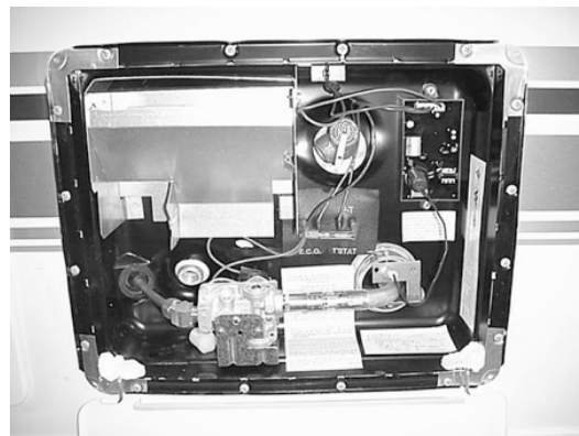
Water Heater Exterior Service Access
