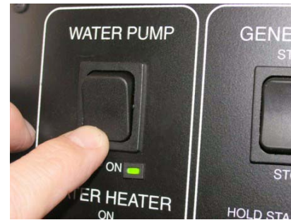
Water Pump Switch
