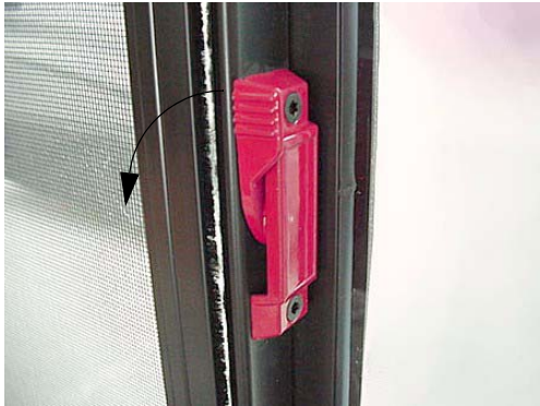
Pull latch outward to slide window open
