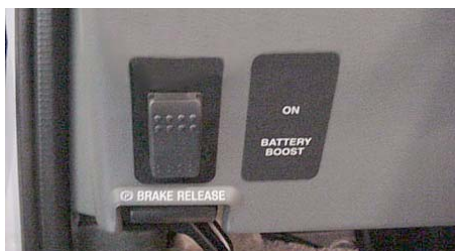
Battery Boost Switch
