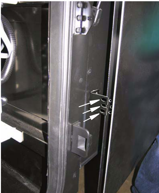
Remove 3 screws from front edge of condenser grille panel in locations shown.
