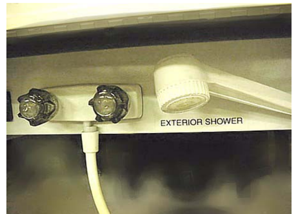
Exterior Shower/Wash Station (typical)
