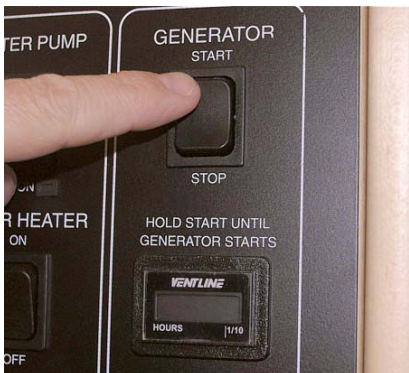
Generator Switch and Hourmeter
