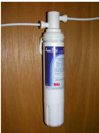
Water Filter Assembly below Galley Sink
