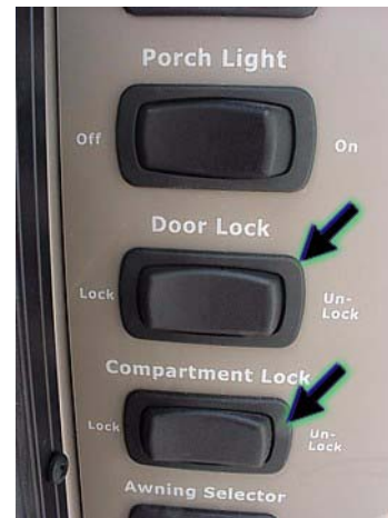
Power Door Locks on entry switch panel
