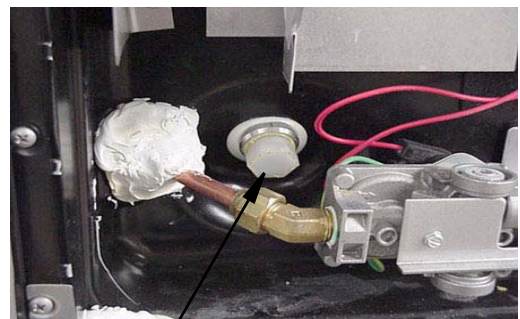
Water Heater Drain Plug Remove with socket
