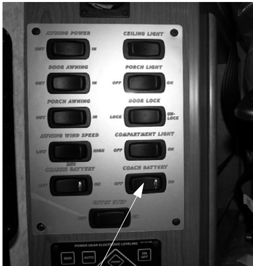
Auxiliary Battery Switch - Typical (Near Entrance Door)
