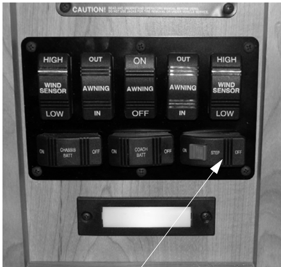
Entry Step Switch (Located near the entrance door)
