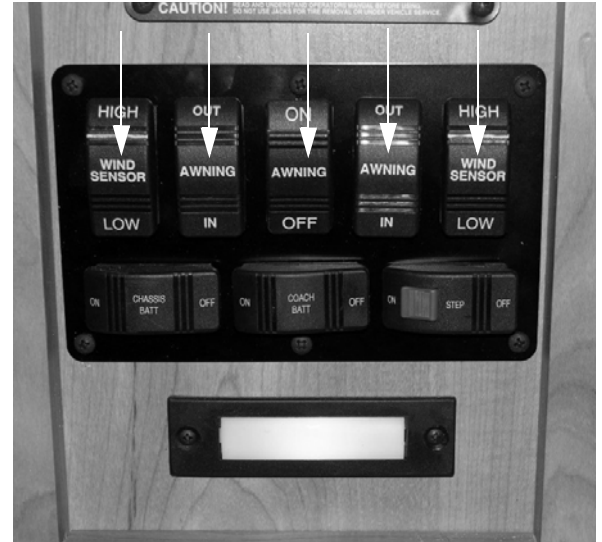
Awning Control Switches - Typical View (Located near entrance door)
