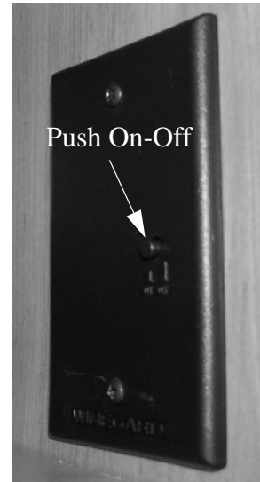
TV Signal Amplifier Switch (Typical View) -Model M39N shown
