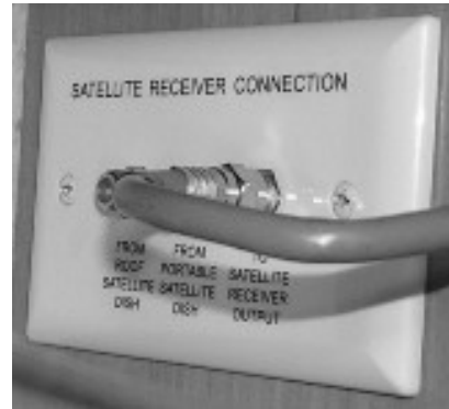
Interior Connection for Satellite Dishes (Located in cabinet near TV) Typical View -Model M39N shown
